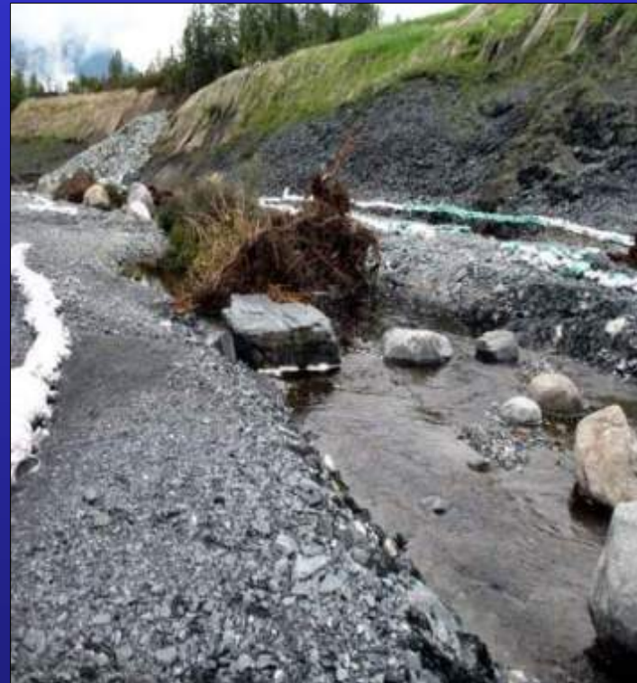
Ketchikan Airport Stream Realignment, AK
