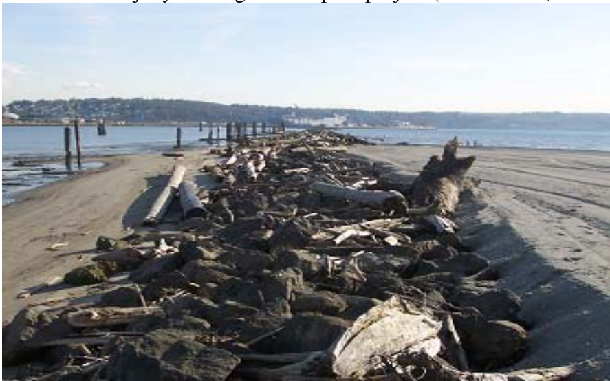
Photo 6: Rock jetty looking south – post-project (March 2007)
