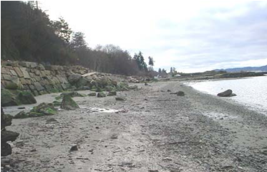
Photo 2: Pre-construction photo on eastern side of proposed enhancement looking west toward derelict tank farm.
